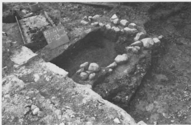
Fig. 8. Svillestener fra stavkirken S:t Stefans nord-vestre hjørne. – Foundation stones for the north-western corner of the stave church.
